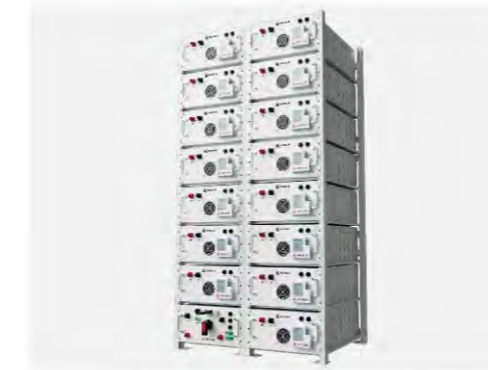
Lithium Battery Energy Storage System
