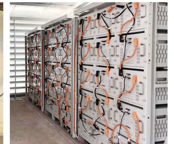
WHC-50KW-Li-430KWH Solar Energy Storage System Location: Freetown, Sierra Leone
